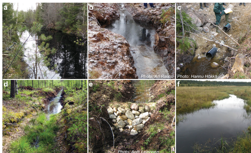
Figure 2. Structures applied in drained peatland forestry to control water quality: sedimentation pond (a), sedimentation pit (b), peak runoff control structure (c), break in cleaning (d), submerged weir (e), and wetland buffer (f).
