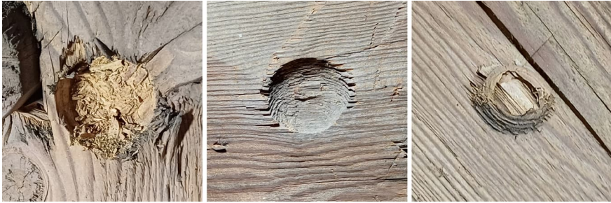
FIGURE 9 Traces of three different types of drill. The trace of a comparatively larger diameter drill (left), the drill mark of a spoon-shaped drill (middle) and the drill mark of a drill with an edge (right)
