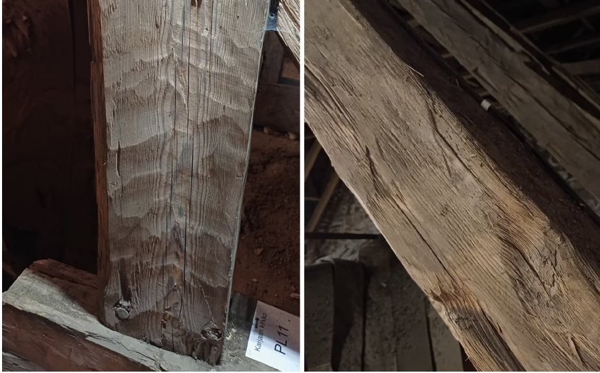
FIGURE 5 Hewing marks on an ashlar post indicate manufacturing by axe (left). The cleaved surface of a scissor beam, in some places, additionally hewn (right) PHOTOS BY FRANZISKA DALHEIMER (2024)
