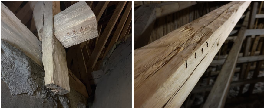
FIGURE 6 Numberings on a sole piece (left) and on a scissor beam (right). Both photographs are taken from below PHOTO ON THE LEFT BY LAURA LAINE (2024), PHOTO ON THE RIGHT BY MIINA TOLONEN (2020)
