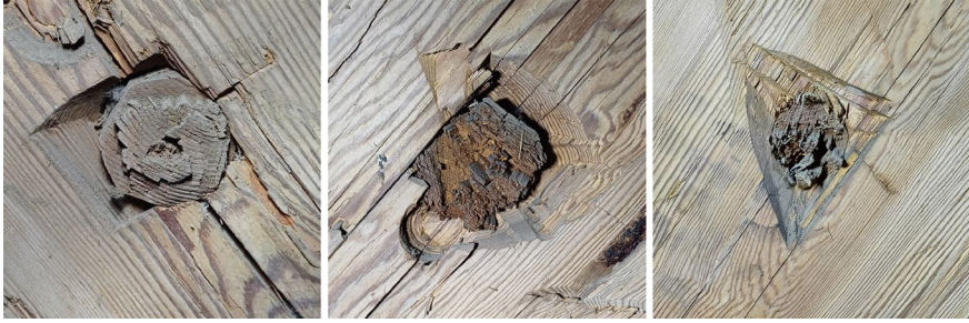
FIGURE 8 The different starting notches made before drilling the dowel holes: a square-shaped starting notch (left), a round-shaped starting notch with rather undefined edges (middle) and a triangle-shaped starting notch (right) PHOTOS BY FRANZISKA DALHEIMER (2024)
