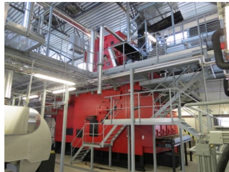
Figure 38: 6 + 5 MW district heating plant in Karjaa, Finland with 1200 m 3 storage. Photo by courtesy of Laatikattila Oy.
