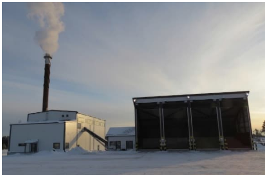
Figure 38: 6 + 5 MW district heating plant in Karjaa, Finland with 1200 m 3 storage. Photo by courtesy of Laatikattila Oy.
