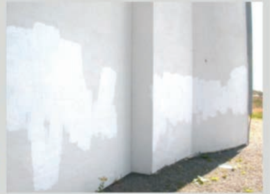
Figure 2.15: Layers of white had been painted to cover the graffiti decoration on the church wall. The layers unfolded stories of the past.
