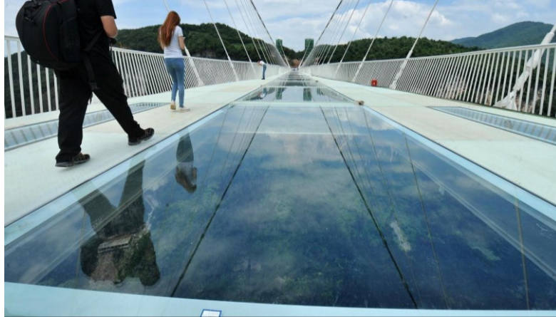
Figure 2.11 Pedestrian bridge with glass deck in Zhangjiajie, China [33].
