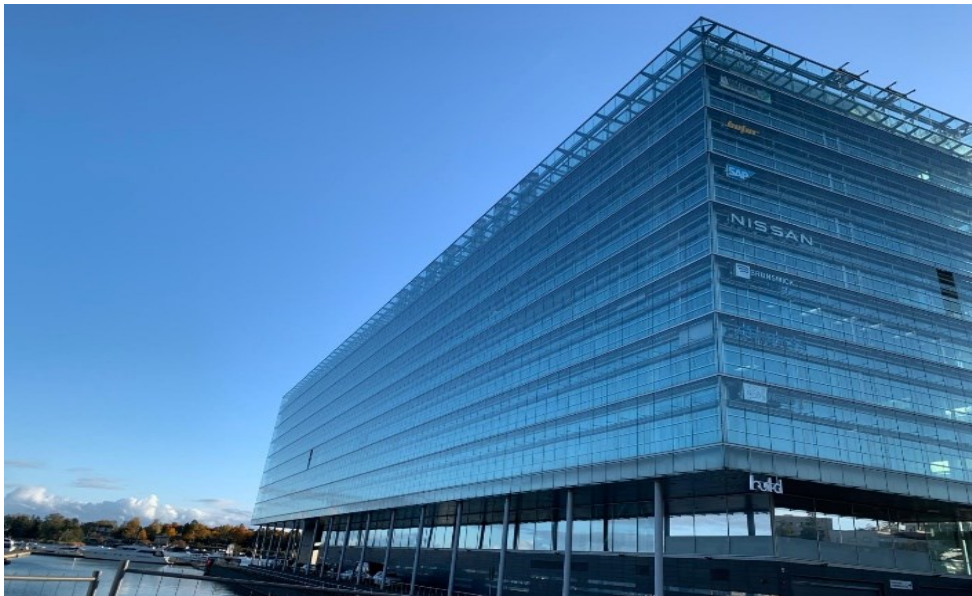
Figure 2.8 Building glass façade in Espoo, Finland.
