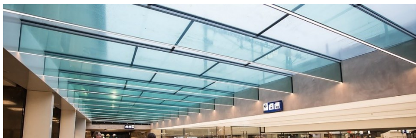
Figure 2.10 Glass structural beams in Eindhoven central railway station, The Netherlands [32].
