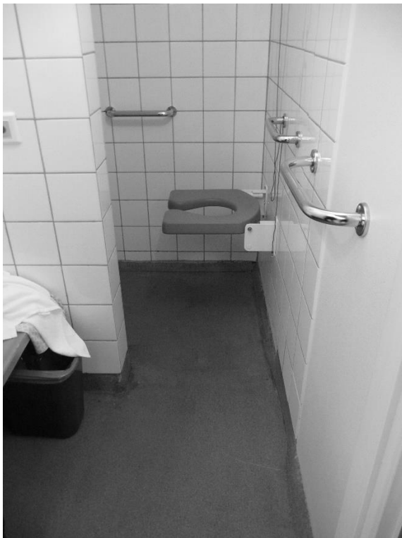
Plate 5. Cramped shower room
