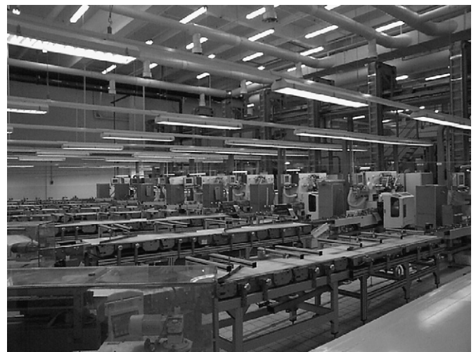
Fig. 1. Test area: packaging room. Note the general diffuse lighting at ceiling level supplying a general uniform illuminance of 400 lux at 1 m above floor level, and the additional task lighting installed parallel to the packaging lines.
