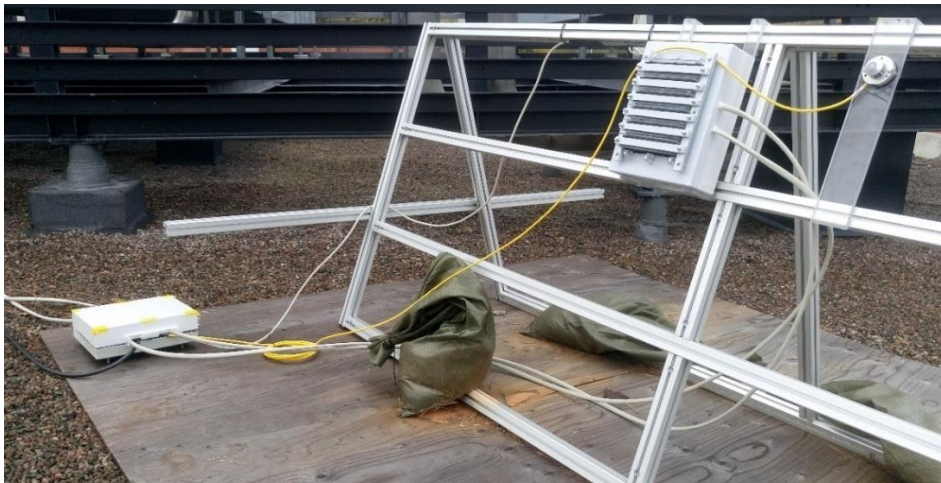
Figure 10. Roof station of the measurement setup. The cell platform is hanging on the stand and the connector terminal is on the plywood on the left.
