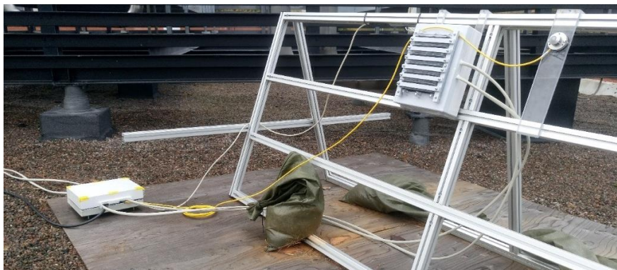
Figure A3. Roof station. The cell platform is hanged to the stand next to the pyranometer. The connection terminal is the grey box next to the stand.
