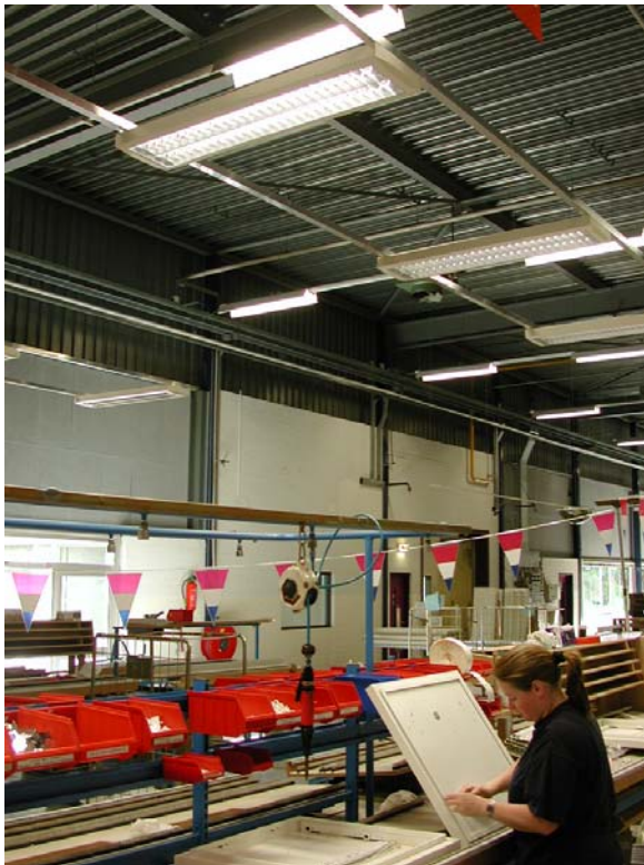
Figure 1. New localised lighting installation. General lighting by white reflector luminaires and localised task lighting by suspended low-brightness luminaires.
