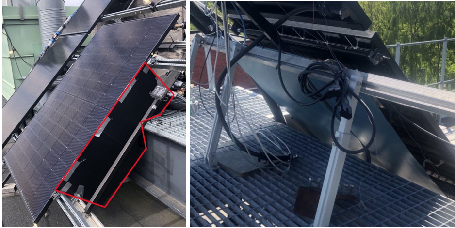
Figure 8: Right) Example of a side panel attached to the PVT. Left) Example of a back panel attached to the PVT.
