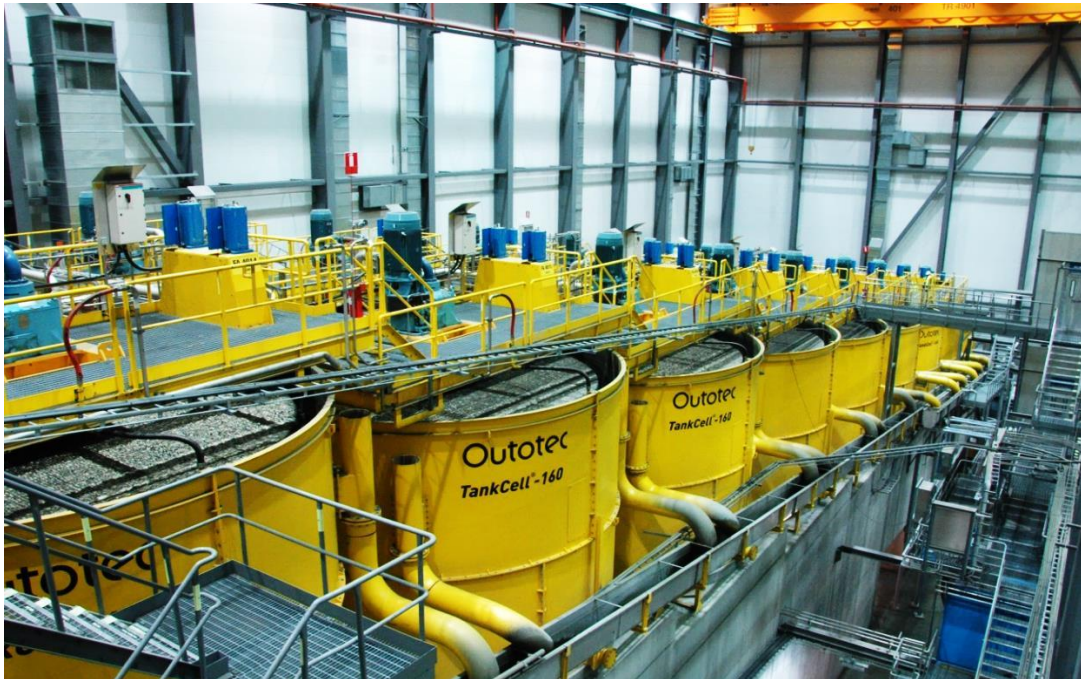
Figure 15: A typical flotation cell tank series forming a bank (Outotec, 2014a)
