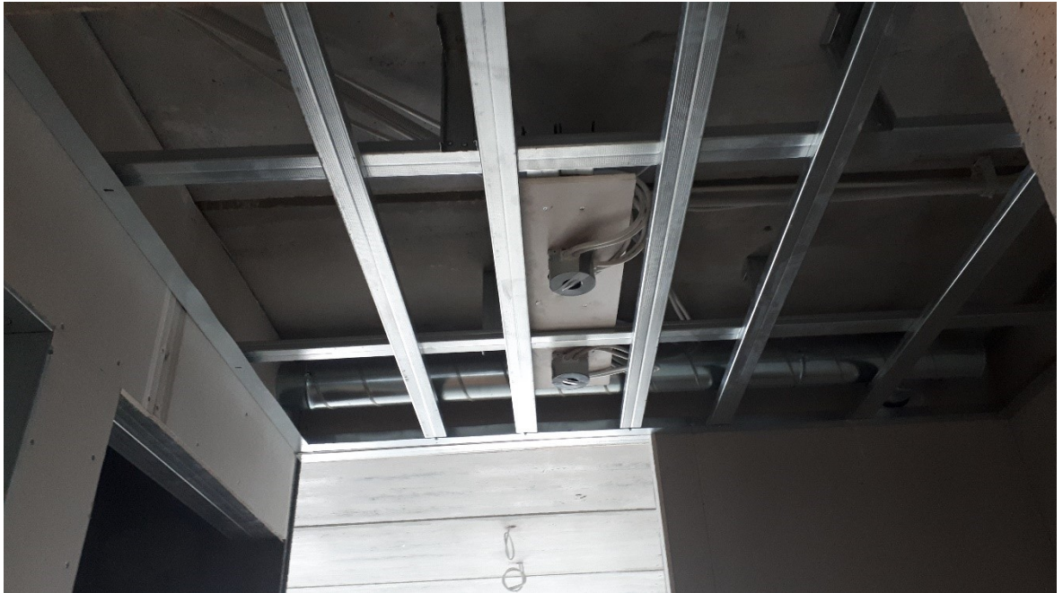
Figure 9: Framework for a gypsum suspended ceiling with electric installments done
