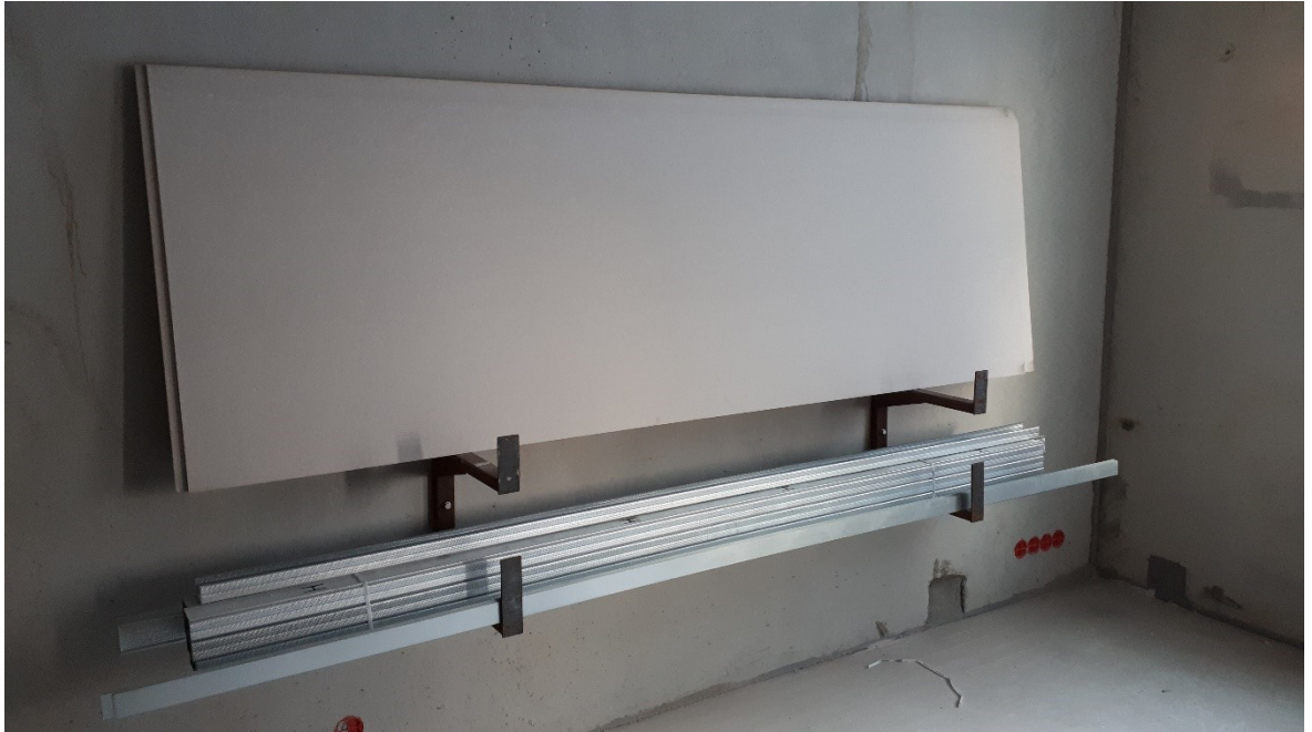
Figure 17: Drywall and frame material wall mount with some materials in it
