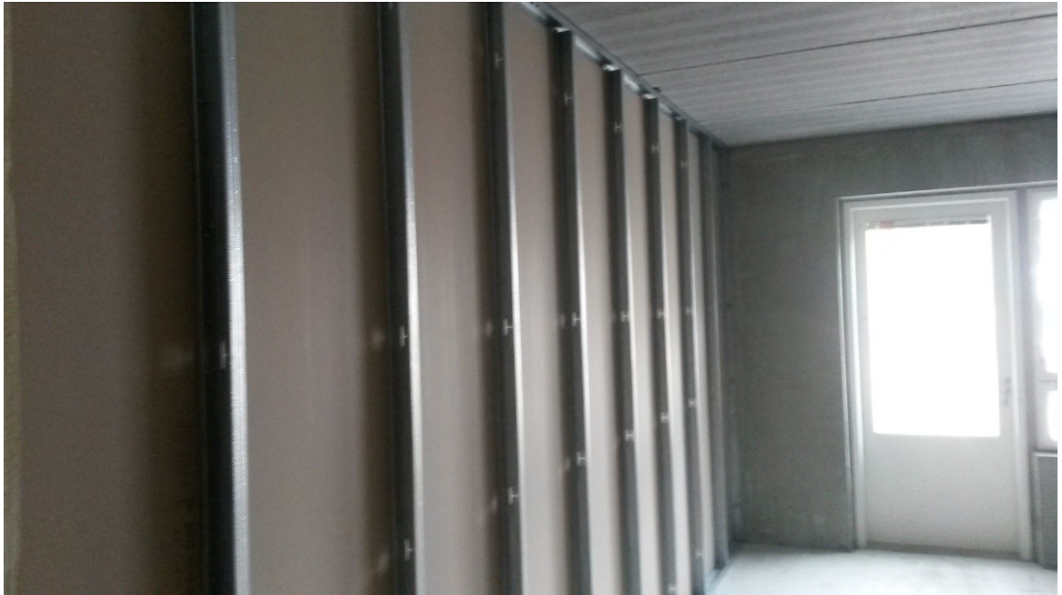
Figure 8: Drywall assembly with steel frame, one side of the sheeting done
