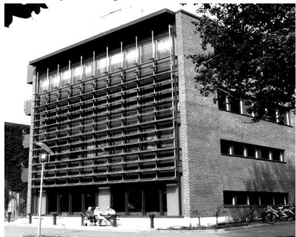
Fig. 2. The south façade of the test building «Valotalo»
